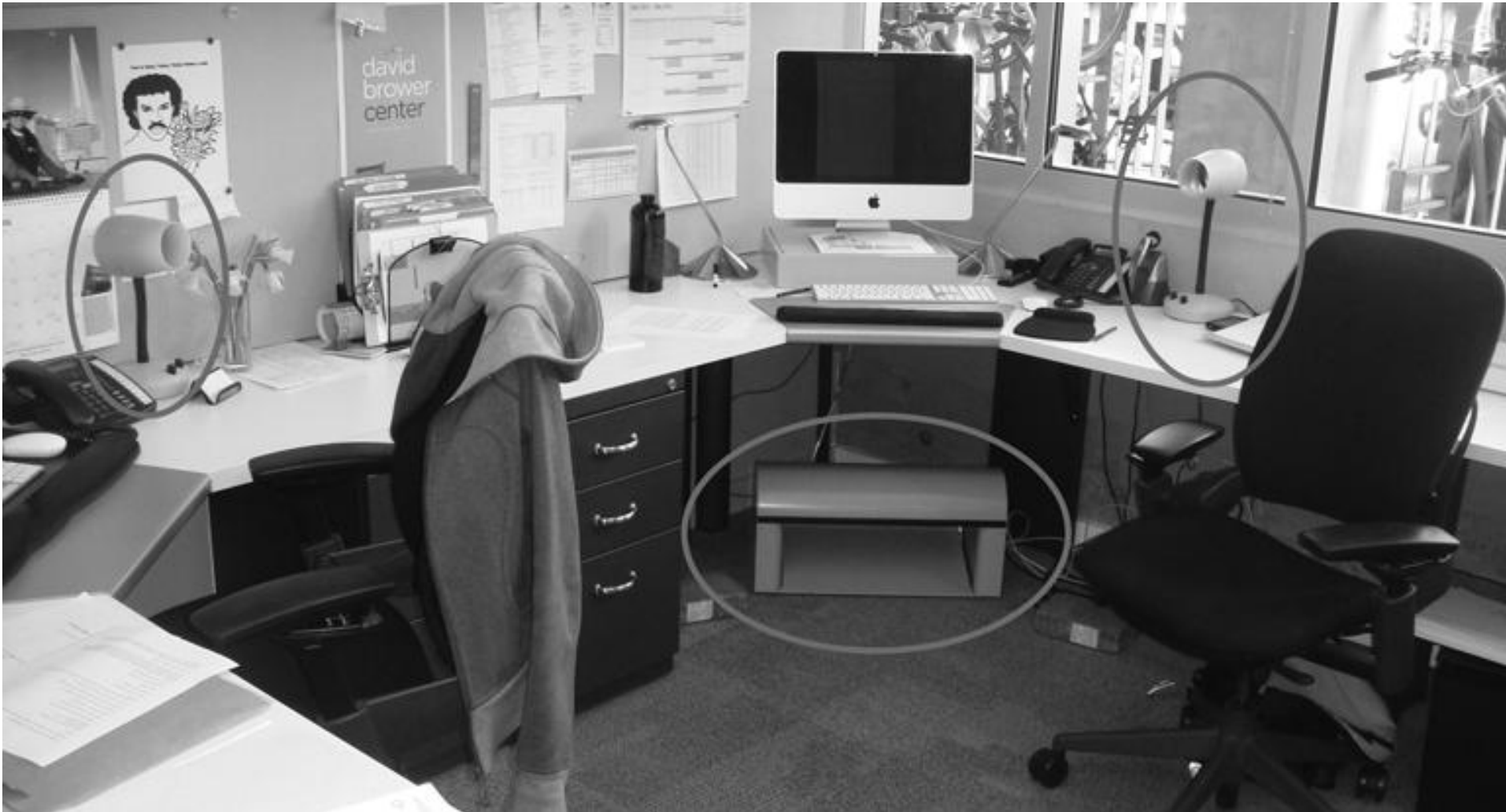
PEC Devices (Fans and a Radiant Foot Warmer) in an Office. Photograph by Ed Arens; courtesy of Center for the Built Environment
